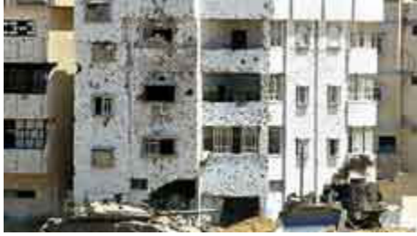
Figure 17. Devastated Building in Gaza
