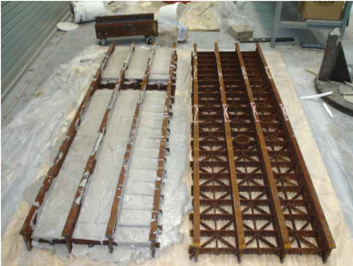
Figure 3-4: Pouring of E-Bond 526 LW Materials to Open Steel Grate Decks.
