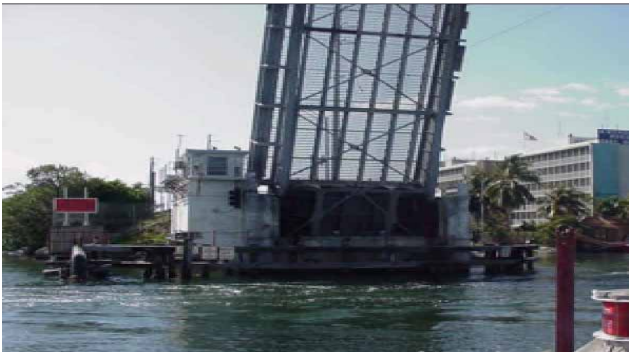
Figure 2-2: Open Steel Grate Deck Systems - Jewfish Bascule Bridge.
